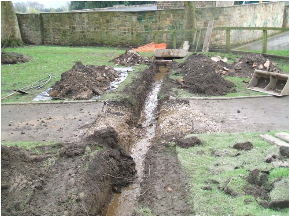
New land drain being constructed at Horsforth Hall Park
