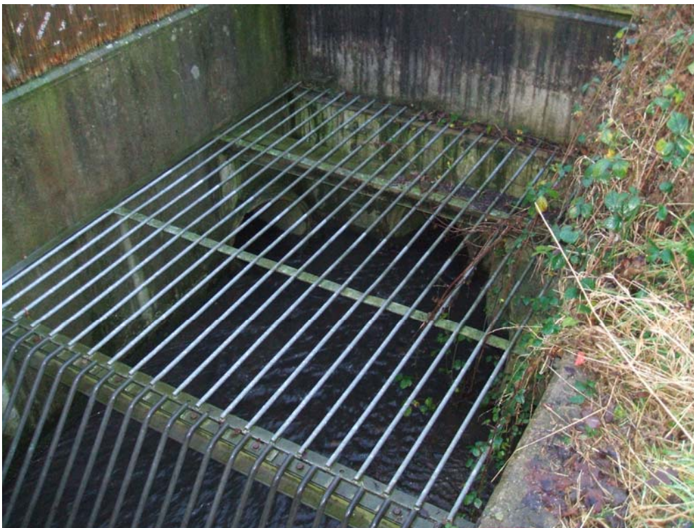
New grid at The Square, Kippax installed by Land Drainage
