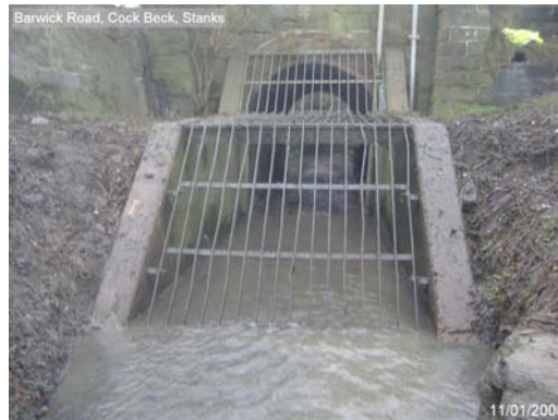
Barwick Road grid on Cock Beck, Stanks, post-fortnightly maintenance on 11 January 2008
